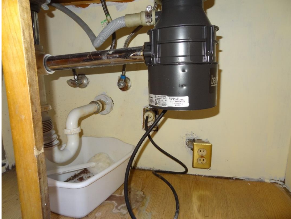
SRC Training and Admin, Building #600-601 - FCA #0322 Description: Electrical outlet missing cover plate under sink. Leaking plumbing fixtures and water damage.
