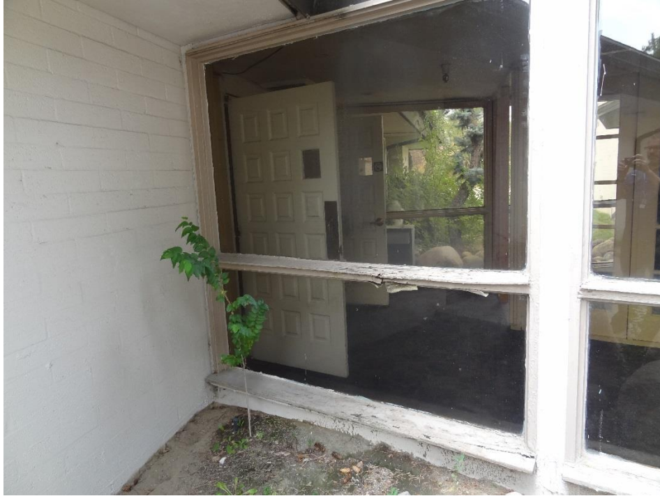
SRC Training and Admin, Building #600-601 - FCA #0322 Description: Missing safety glazing and damaged window framing.
