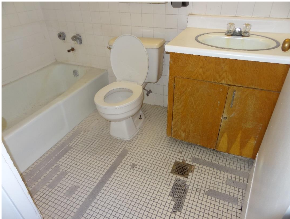
SRC Training and Admin, Building #600-601 - FCA #0322 Description: Typical restroom finishes.
