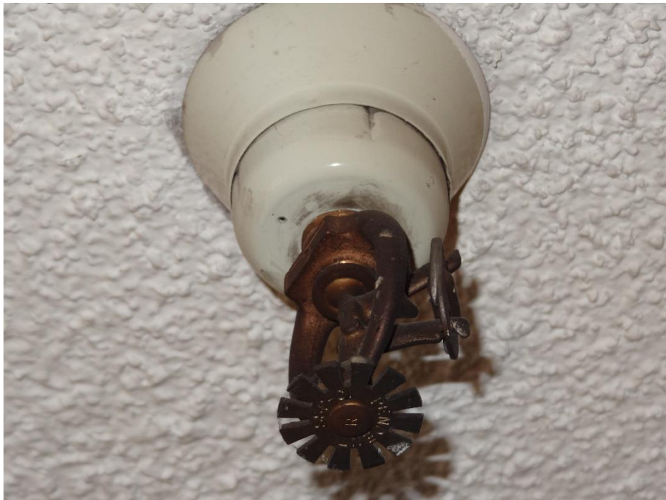
SRC Training and Admin, Building #600-601 - FCA #0322 Description: Antiquated fire sprinkler head.
