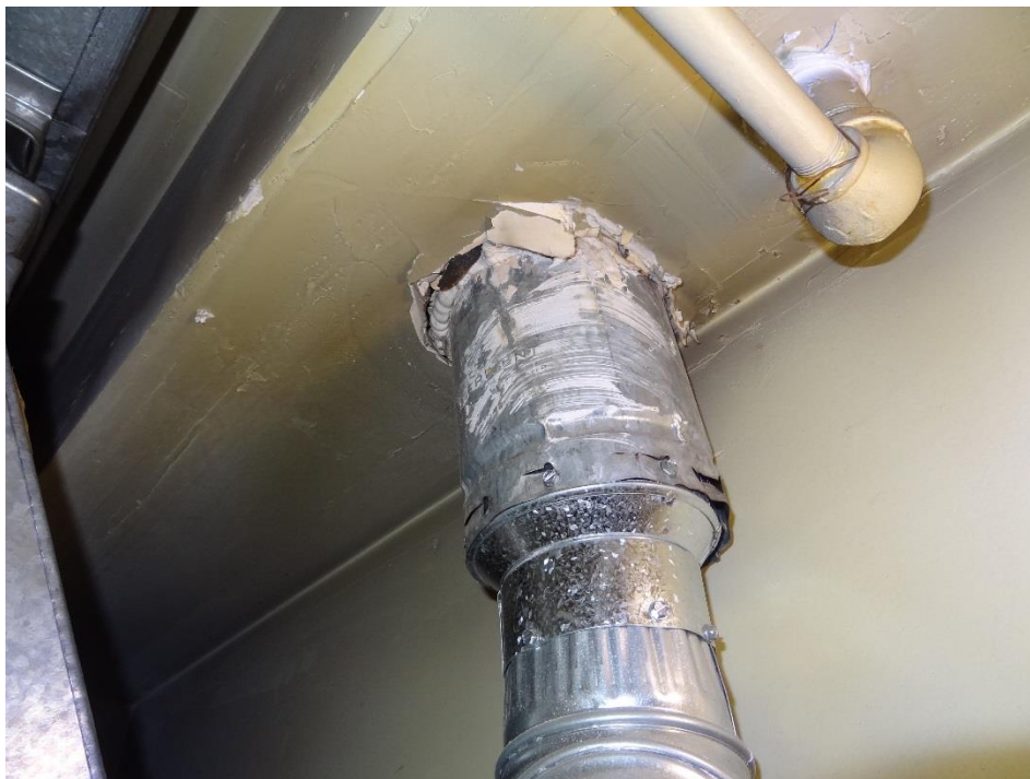
SRC Training and Admin, Building #600-601 - FCA #0322 Description: Flue vent with improper installation.
