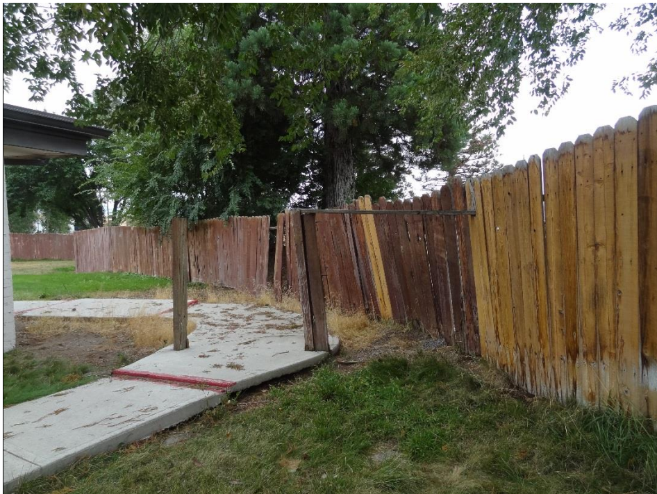
SRC Training and Admin, Building #600-601 - FCA #0322 Description: Damaged sidewalks and fencing.
