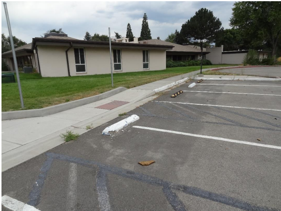
SRC Training and Admin, Building #600-601 - FCA #0322 Description: ADA parking spaces and signs removed.
