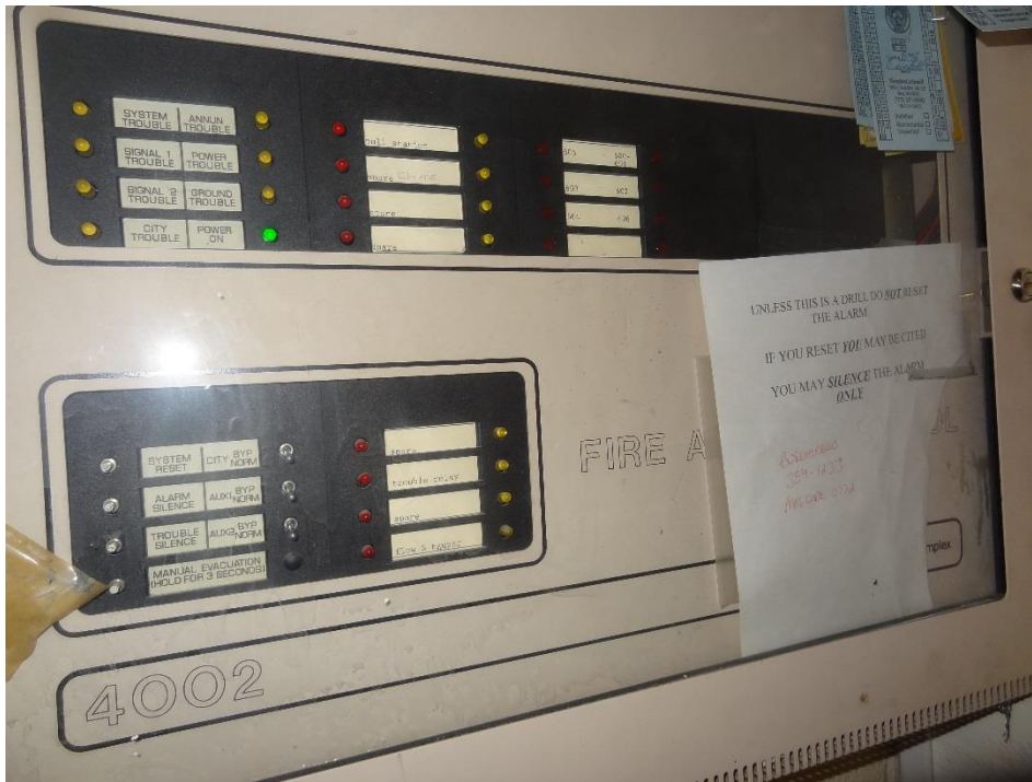
SRC Training and Admin, Building #600-601 - FCA #0322 Description: 27 year old fire alarm system.
