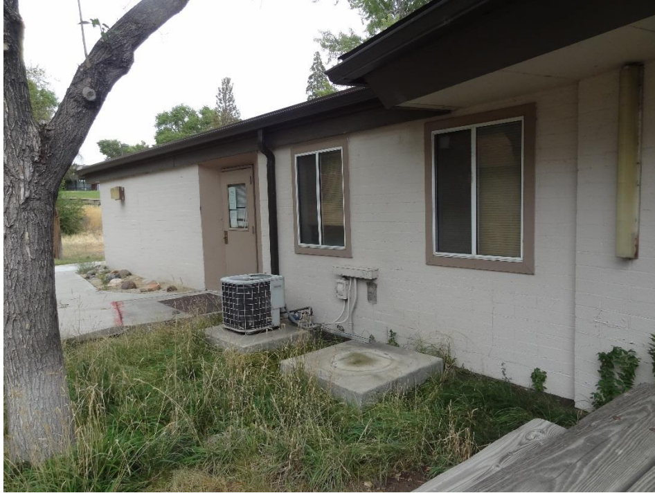
SRC Training and Admin, Building #600-601 - FCA #0322 Description: Missing air conditioner.
